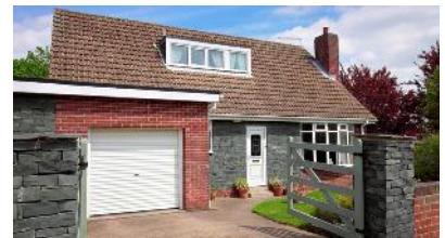
Roller Garage Doors
